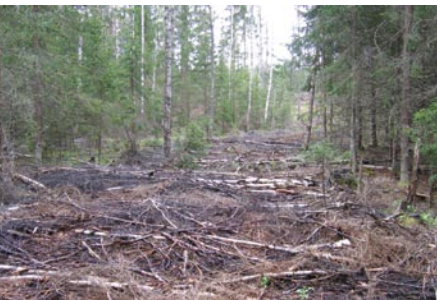
A twig mat made of birch - the cheapest method to minimise damage to the ground and to the watercourses
