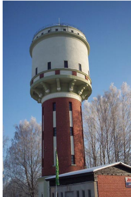
Water storage tower
