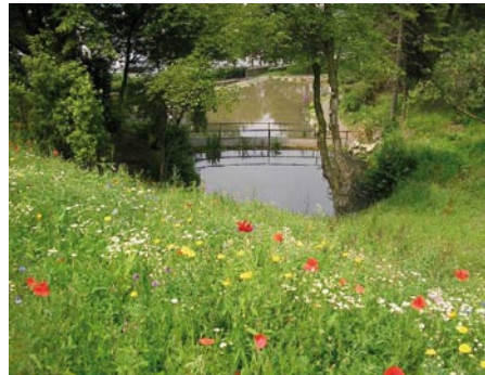
Broadfield Pond after restoration
