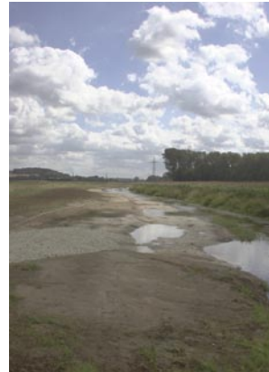
River Else - remodelling of riverbanks
