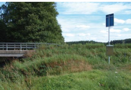
Flow metre station with solar cell
