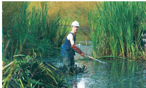
MWH PROCESS ENGINEER PAUL FLETCHER HELPS CLEAN THE SANKEY CANAL
