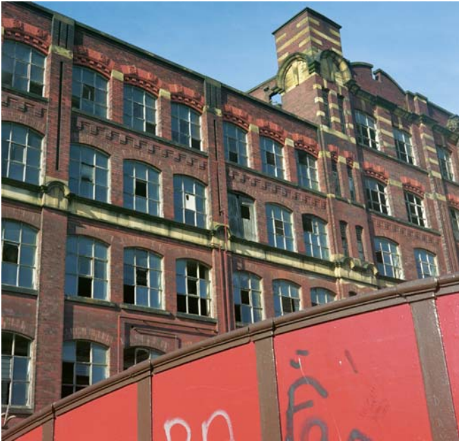
ROYAL MILLS IS AT THE HEART OF A MULTI-MILLION POUND REGENERATION SCHEME
